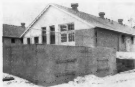
Fig. 1—Photograph showing the construction of the manure pit.
